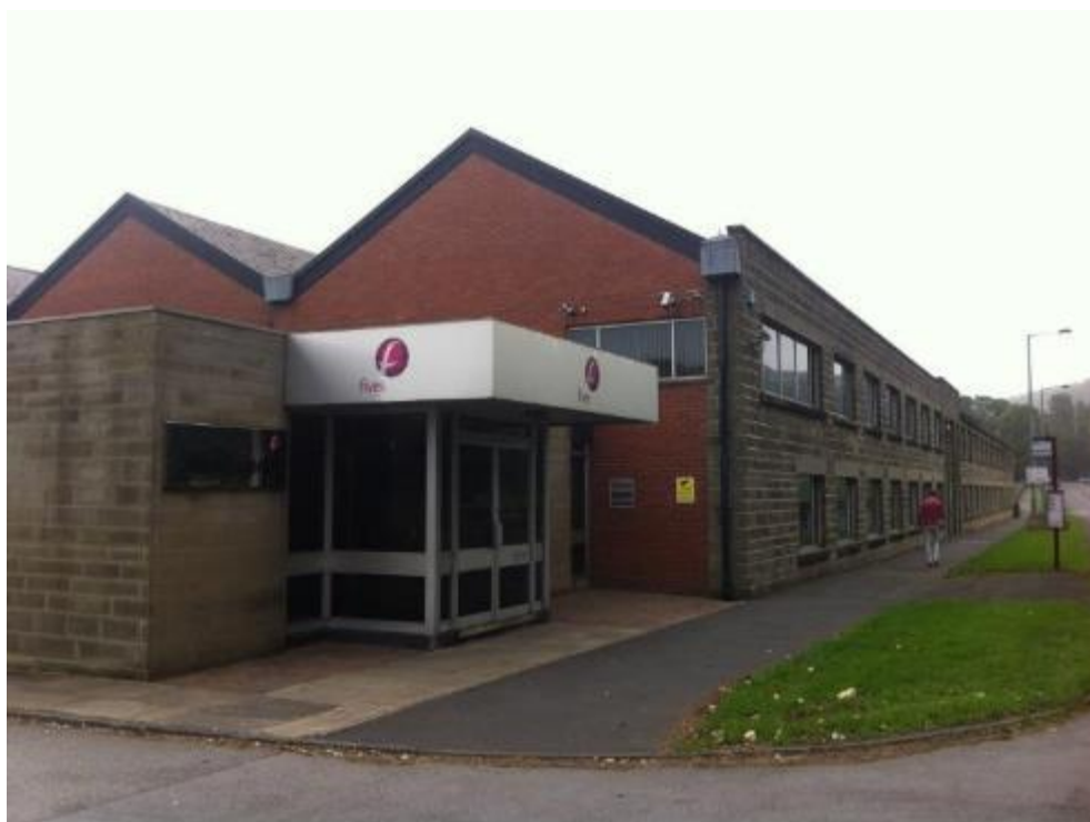
Eastburn Works, Skipton Road, Eastburn
